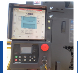
Operator's Control Station
